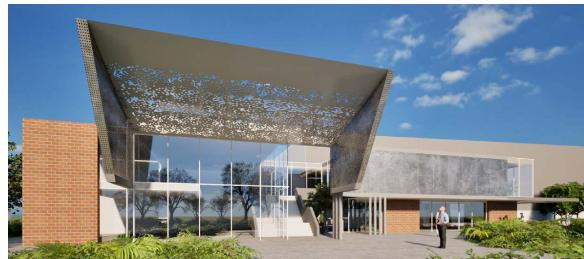
**Figure 159** Rendered impression of an indicative building with heat resilient design solutions using light-coloured materials for facade and hardscaping as well as canopy structure that extends beyond building footprint to shield glazing from heat load, reflect light and release heat at night.
