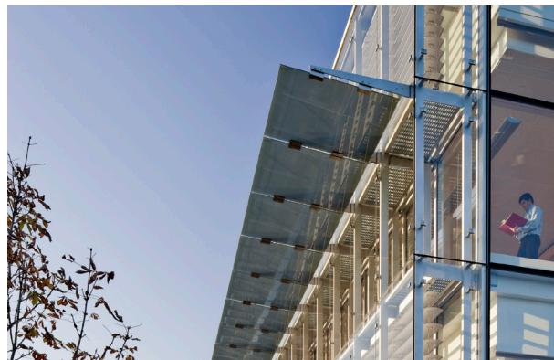
**Figure 162** Example of passive solar building design utilising sun-shading device to manage daylight into office space and reduce reliance on electrical lighting during daytime.
