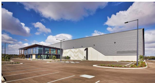
**Figure 130** Example of design solutions to break down long façades via juxtaposition of different functional programs and built forms.
